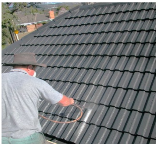
THIRD COAT - CRC MEMBRANE OR SUPA COOL MEMBRANE
