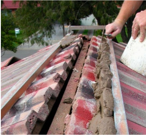
RE BED WITH NEW MORTAR
