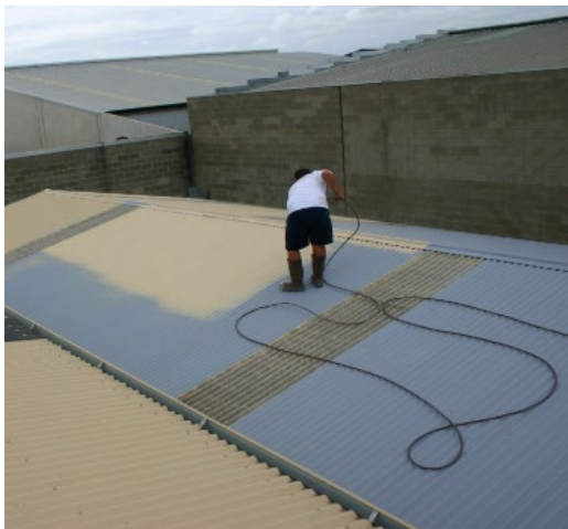
SECOND COAT - CRC MEMBRANE OR SUPA COOL MEMBRANE
