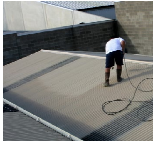
THIRD COAT - SECOND MEMBRANE COAT - CRC OR SUPACOOOL
