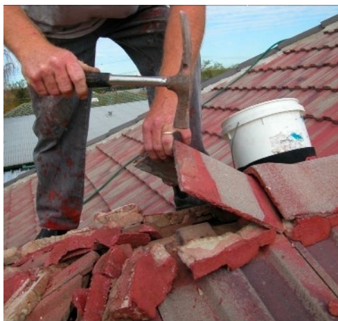
REMOVE RIDGE CAPPING & DAMAGED BEDDING AS REQUIRED
