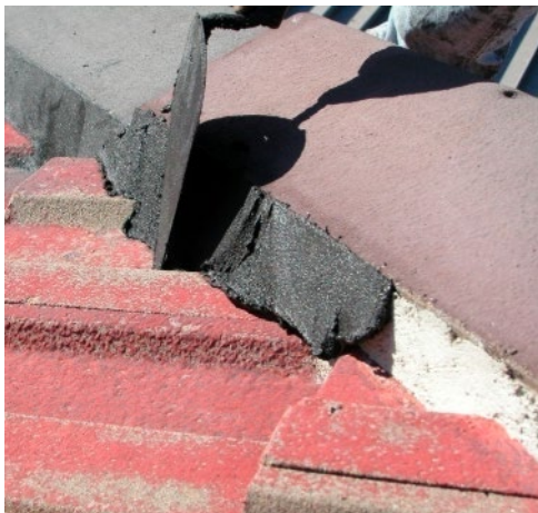
RE POINT WITH FLEXIBLE POINTING
