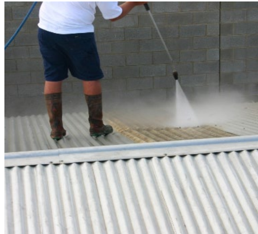
PAINT WILL NOT STICK TO A SURFACE THAT IS DIRTY!
