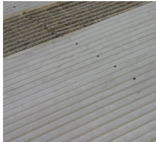
ROOF IS DULL, DIRTY & FADED
