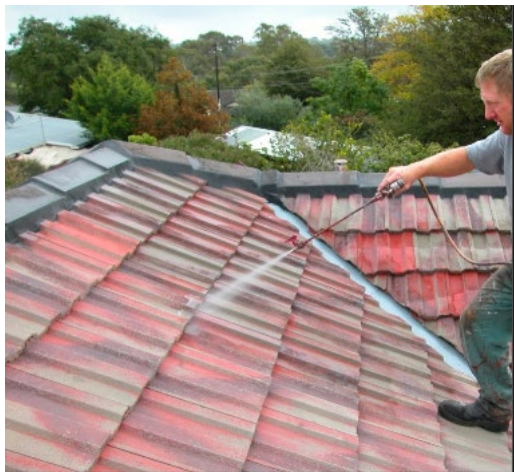
FIRST COAT - ACRYLOC MOULDRID, SLOWS FUTURE MOULD GROWTH
