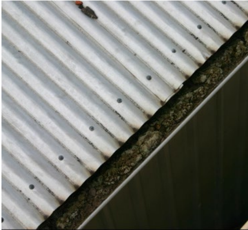
ROOF IS DULL, DIRTY & FADED
