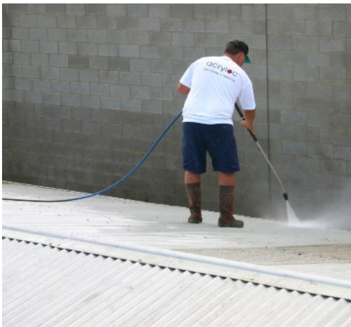
PAINT WILL NOT STICK TO A SURFACE THAT IS DIRTY!
