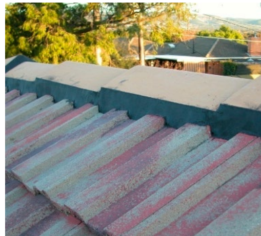
REPAIRS COMPLETE & RINSE OFF ROOF TO REMOVE DUST, READY FOR COATINGS
