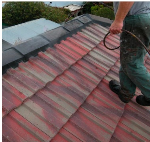
SECOND COAT - ACRYLOC PRIMERBOND ROOF RESTORE, ESSENTIAL FOR ADHESION!
