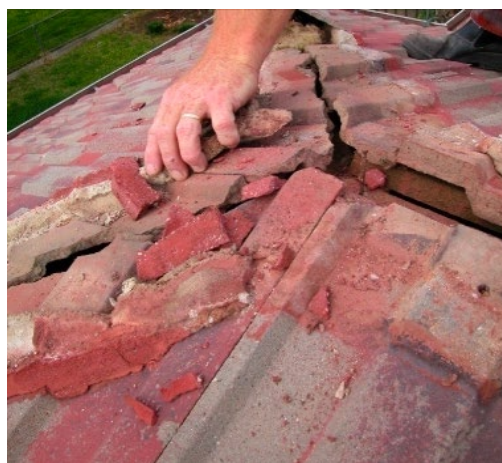
REMOVE RIDGE CAPPING & DAMAGED BEDDING AS REQUIRED
