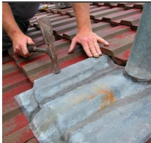
REPAIR FLASHINGS
